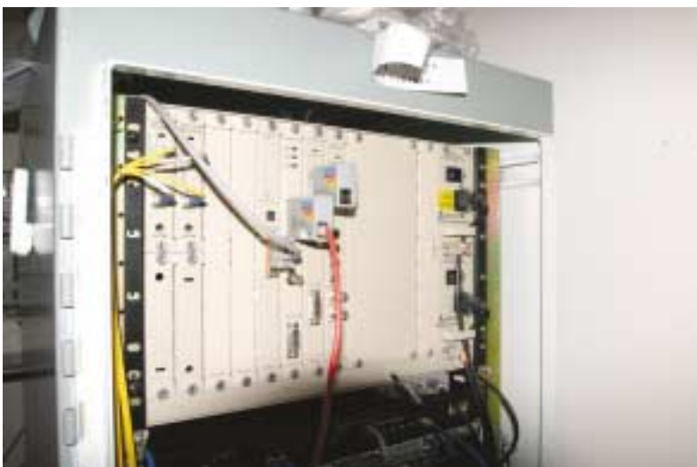
Close-up of PremNet5000 chassis which was replaced by a Redundant Ring Ethernet Switch.
