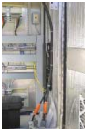
Equipment enclosure with various communications equipment. The TC3720 Redundant Ring Switch is mounted vertically on the right side.
