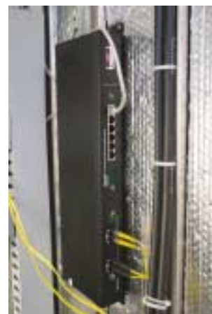
Equipment enclosure with various communications equipment. The TC3720 Redundant Ring Switch is mounted vertically on the right side.
