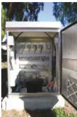
Equipment enclosure with various communications equipment. The TC3720 Redundant Ring Switch is mounted vertically on the right side.
