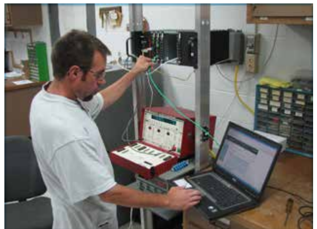
NIPCO Technicians only require a laptop to perform JumboSwitch network health/alarm checks and reconfigurations.
